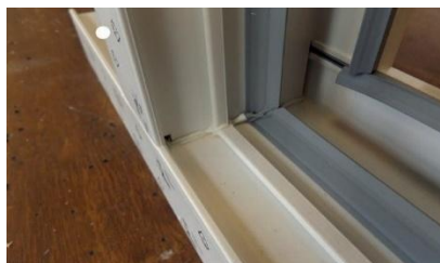
Figure 25: Butt-welded mullion, rebate seal (AD) Figure 25 b: Butt-welded mullion center seal (MD)
